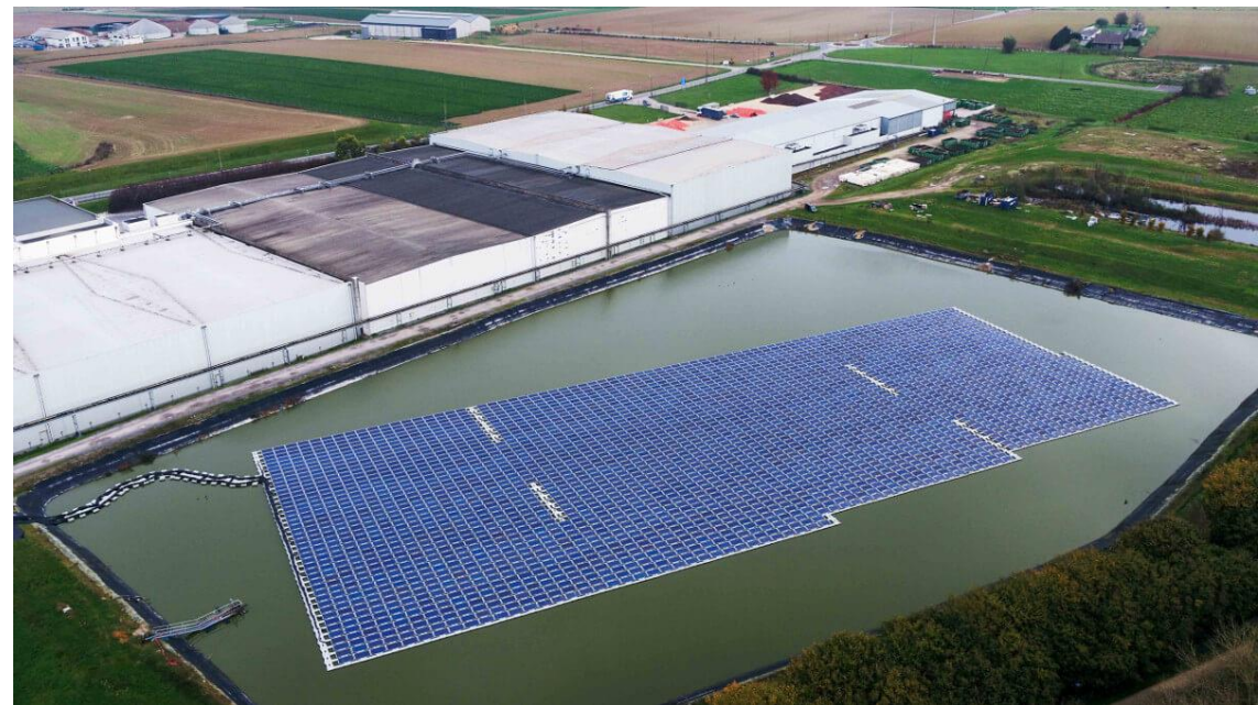
1 MW floating plant Hesbaye Frost, Perpetum
